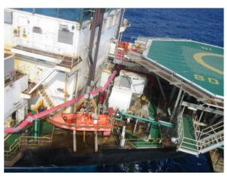
Several valves of a line system on an oil platform were damaged. The problem was abrasion caused by the transportation of sand and sea water. The damages were repaired with the help of Ceramium, pasty.
